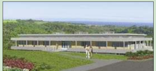
Construction has started on a combination herbarium, library, educational, research and conservation center at National Tropical Botanical Gardens. Courtesy Dean Sakamoto Architects LLC.
